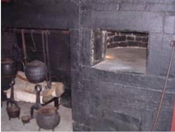
The fireplace shown above is located in the Dana House's kitchen. The hearth still retains its crane and cooking implements. The opening to the right of the hearth is a beehive oven.
